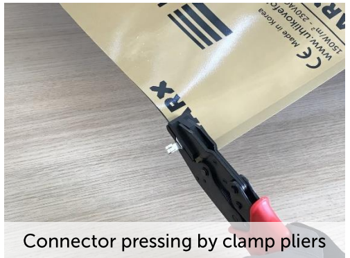
Important is exact connector place
