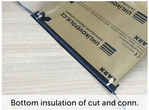
Pressing power cables in connector
