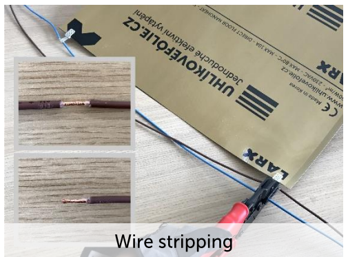
Connector pressing by clamp pliers
